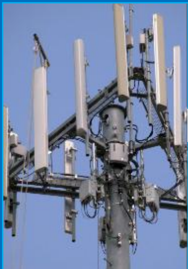
Conventional separate 2 power cables and 4 F/O cables supporting 1 RRU
